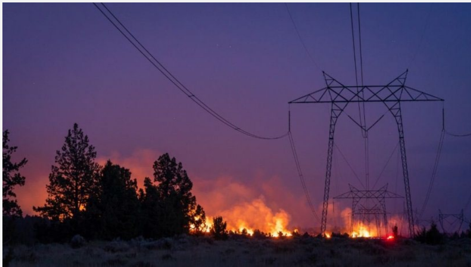
Figure 33: Wildfires and Electrical Infrastructure 60
