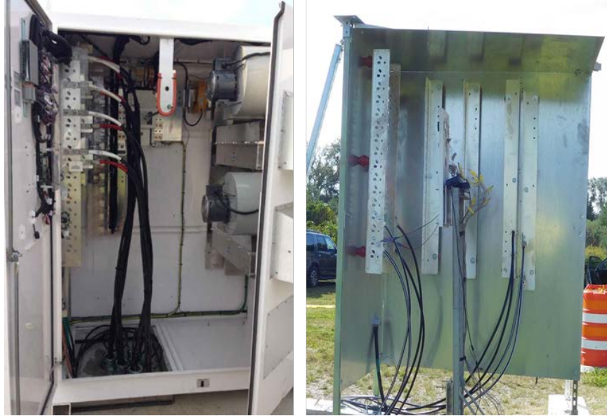
Figure 2-16 Image of an inverter cabinet used as a reference (left) and the mocked-up assembly (right)
